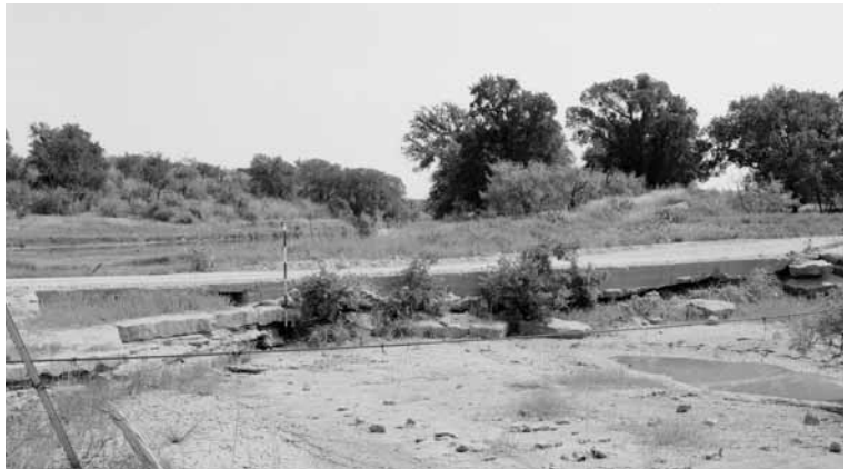
THIS 1989 PHOTO is of a bridge built from 1936-41 as part of a Works Progress Administration (WPA) project in Coleman County, Texas. Many Americans saw such projects as helpful, without considering their high cost and the corruption that plagued the program.
